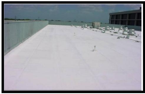
The above pictures show CoverCoat 840 CP over a granulated Modified Roof System.
