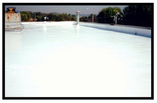
The above pictures show CoverCoat 840 CP copolymer rubber roof coating over an EPDM Roof System. The CoverCoat 840 CP coating creates a monolithic membrane that not only waterproofs the roof but also creates an attractive, highly reflective surface.
